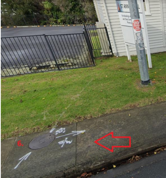
7. SW MH LID, 3.87m RL, 3.89m DEM AUK1946, 1755649,5935123 (on kerb)
