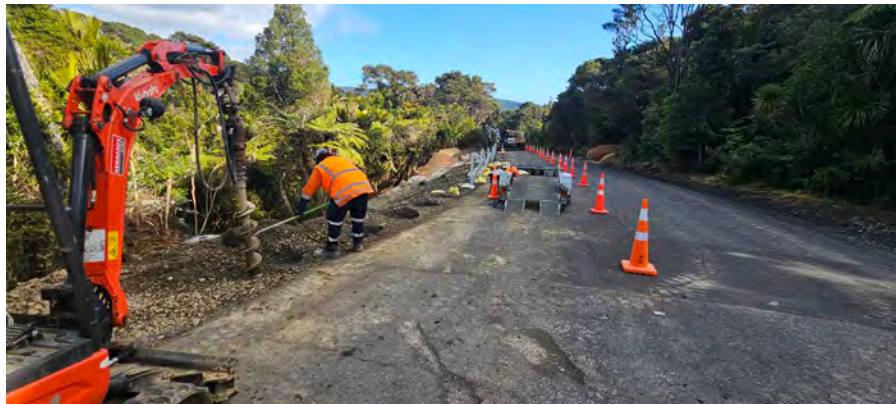
Block retaining wall almost complete
