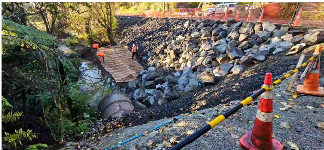
Slip repair underway on Yelash Road
