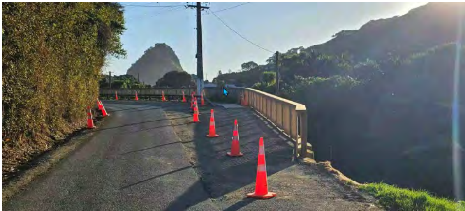
Slip repair on Glenesk Road
