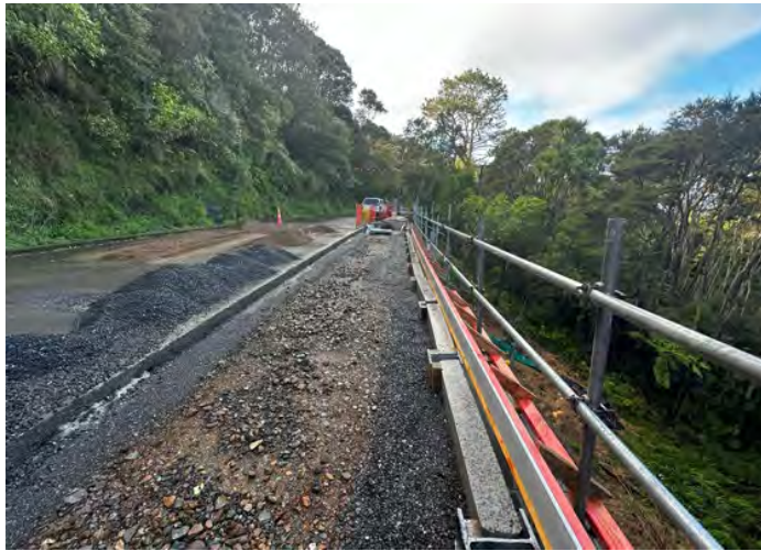
Retaining wall constructed at Titiangi end of Scenic Drive.
