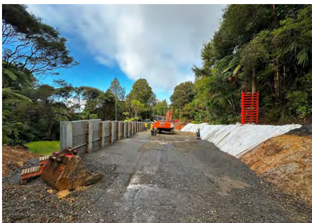
Works progressing, with backfill and culvert works.
