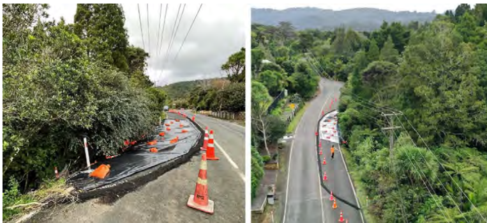
Slip repair to be started in August on Te Henga Road
