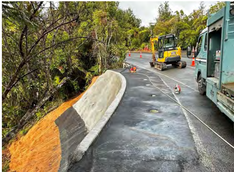
Scenic Drive, Auckland City Look-out slip repair, soil nail wall complete.
