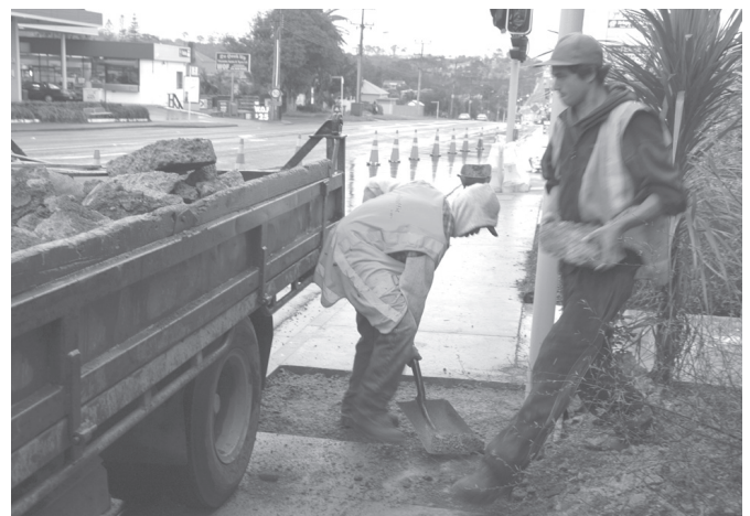
Footpath improvements, Glen Eden
