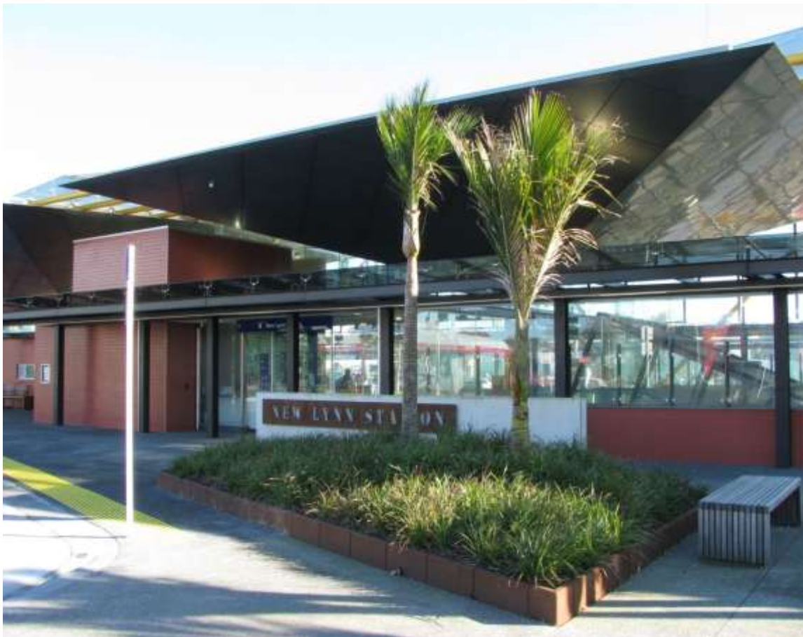
New Lynn Station, an example of a multi-modal transport interchange catering for rail, bus, car, cycle and walking modes
