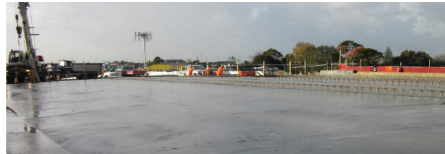
Photo centre: Ellerslie Panmure Highway bridge deck pour completed.
