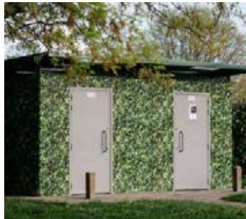
Permanent public toilets
