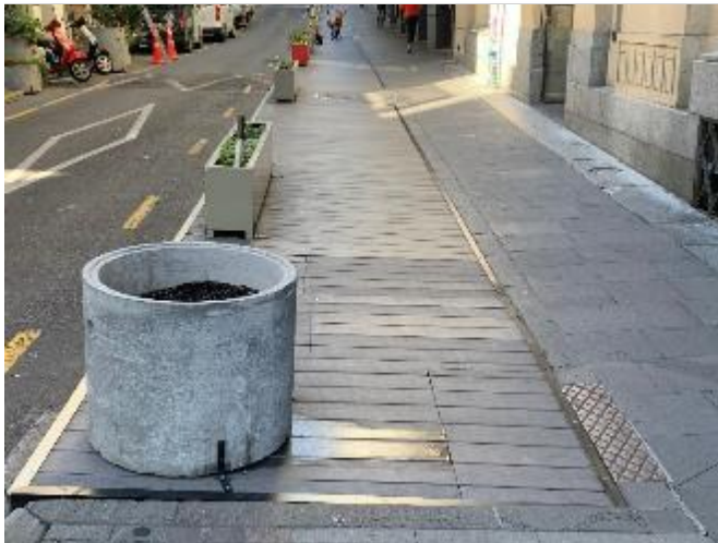
Figure 2.7 Example flush footpath extension - High Street
