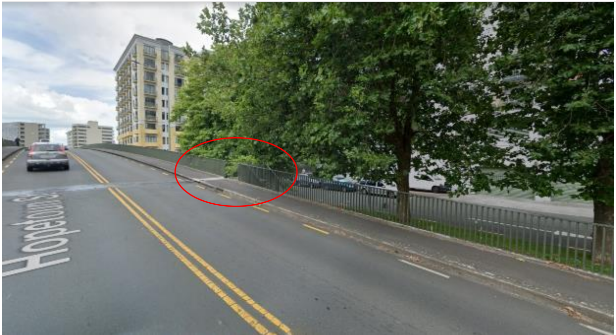
Figure 2.5 Stair access to southern side of Hopetoun Street bridge
