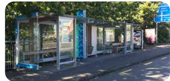
GOOD QUALITY ON-STREET BUS FACILITY AT SYMONDS ST
