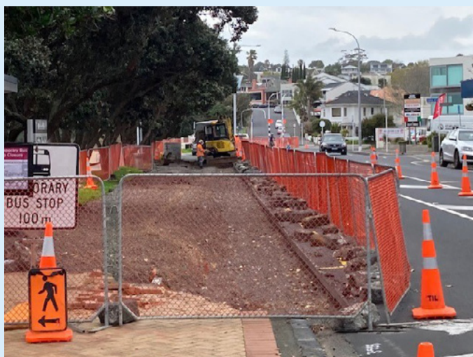
St Heliers project gets back underway at Alert Level 3
