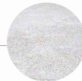
Lightly exposed aggregate concrete pile finish.
