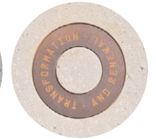
Sandblasted concrete surface with ground pattern and steel disc inserts reflecting the underlying geology & fossil fields under the boardwalk.
