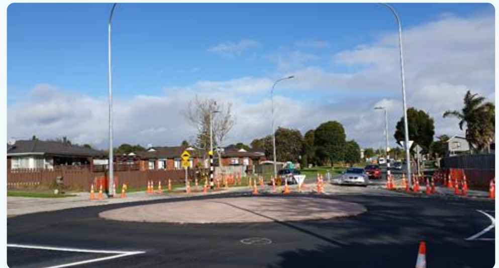
New roundabout constructed at intersection of Bucklands Beach and Sunderland’s Roads
