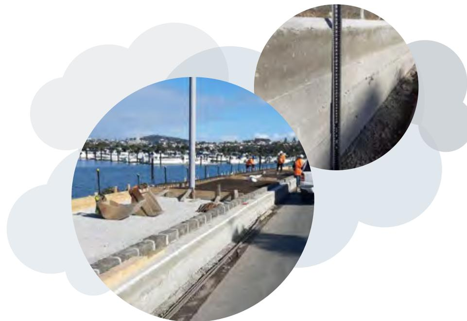
**FIGURE 10: AT HAS RAISED THE HEIGHT OF THE TAMAKI DRIVE SEAWALL TO IMPROVE RESILIENCE TO SEA LEVEL RISE**
