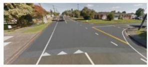
This is like a speed table but it covers an entire intersection - with ramps at each entry point. The intersection is raised to the level of the footpath - making it easier for pedestrians to cross.
