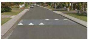
Speed humps are shorter and more rounded than speed tables and are also designed to slow vehicle speeds. The white arrows, and sometimes signage, make drivers aware of the speed hump.
