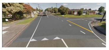
This is essentially a raised table, which covers an entire intersection – with ramps at each entry point. The intersection is raised to the level of the footpath – making it easier for vulnerable road users to cross.
