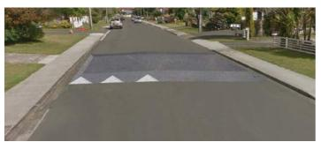
A speed table is a raised section of the road, with ramps on each side, that aims to slow vehichles to a safe speed. The white arrows, and sometimes signage, make drivers aware of the speed table.
