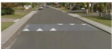
Speed humps are shorter and more rounded than speed tables but are also designed to slow vehicle speeds. The white arrows, and sometimes signage, make drivers aware of the speed hump.
