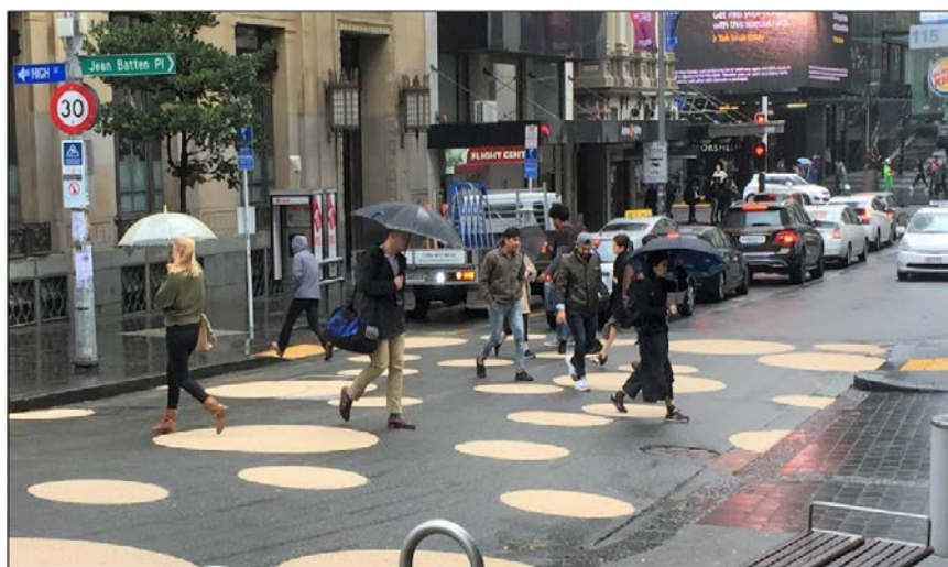
Figure 1: Prior to colour (source safety audit, TES)
