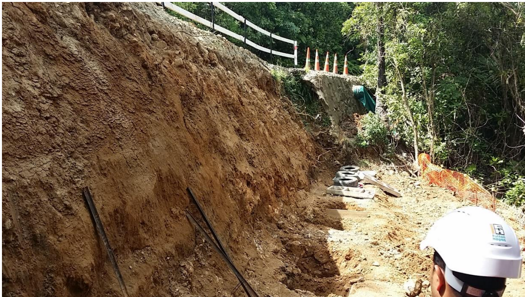
Building a retaining wall to stabilise the Road in Windy Canyon
